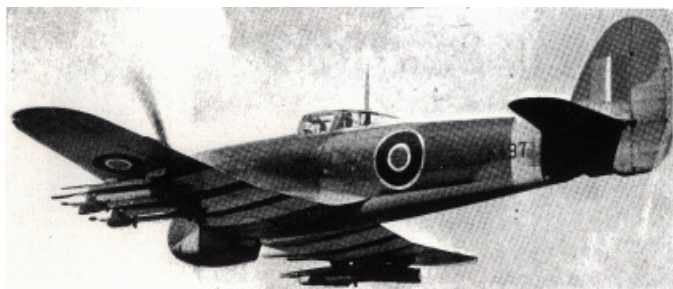
The Hawker Typhoon IB Rocket Fighter (Napier Sabre IIA engine).
